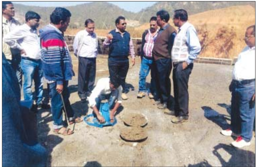
Testing at Telengiri Medium Irrigation Project
