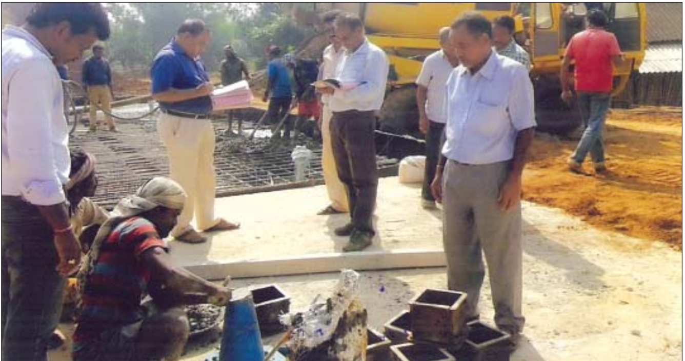
Slump & Cube Testing at Subarnarekha Irrigation Project
