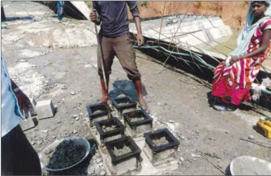
Testing at Telengiri Medium Irrigation Project
